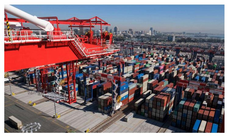
LBCT is a fully automated container terminal and normally has among the lowest rail container dwells and truck turn times in the LA-LB port complex. Photo credit: Ringo Chiu / Shutterstock.com.
